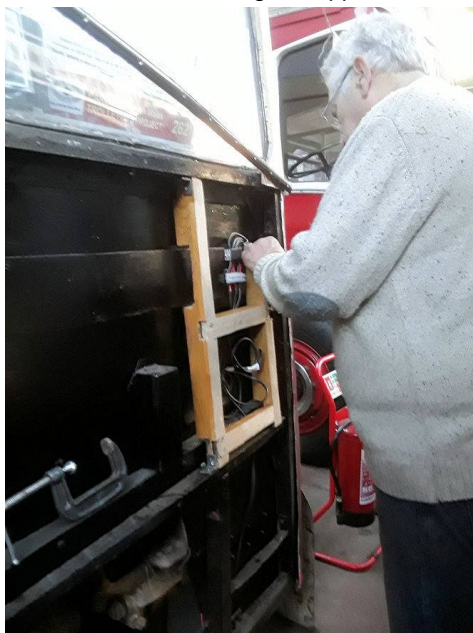
Bob Heatley fitting new under skin timber framing. [Keith Walker]
